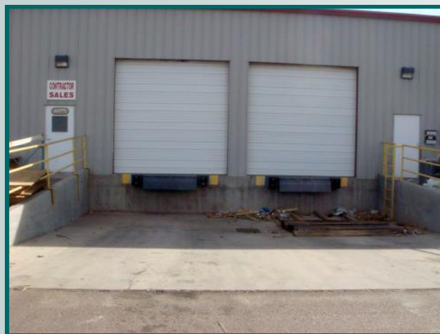
Loading Dock (well)
